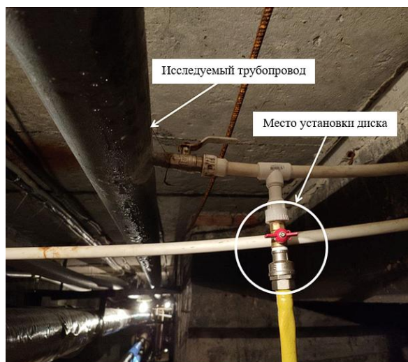
Fig. 7. Photograph of the installation location of the disk on a steel pipeline
